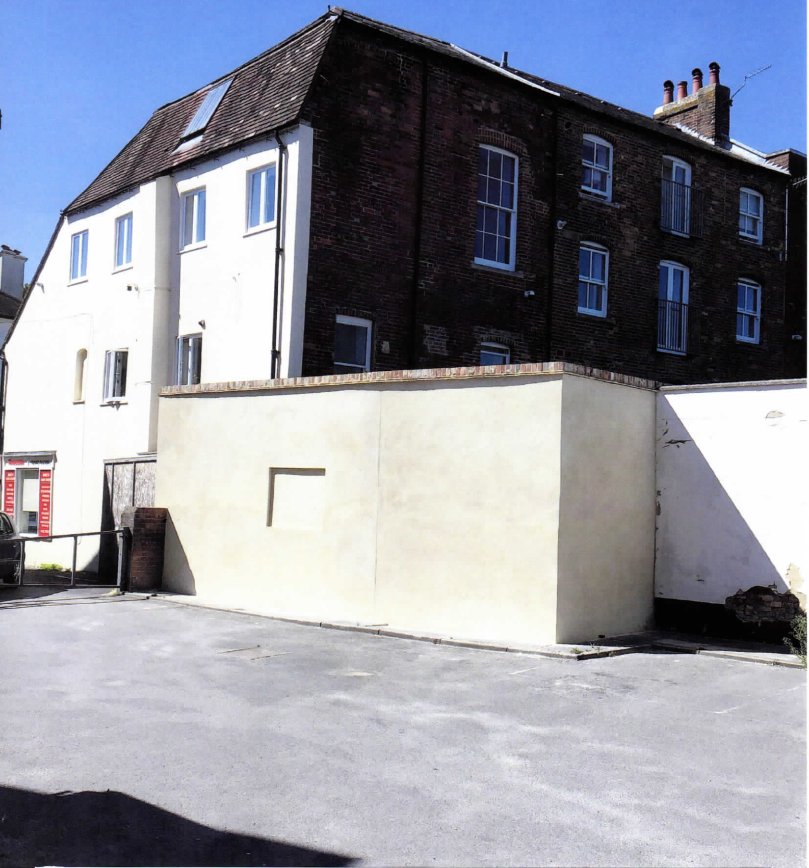
View from proposed beer garden looking towards the flats 6a, 6b, 8, 8a & 8b West Borough
